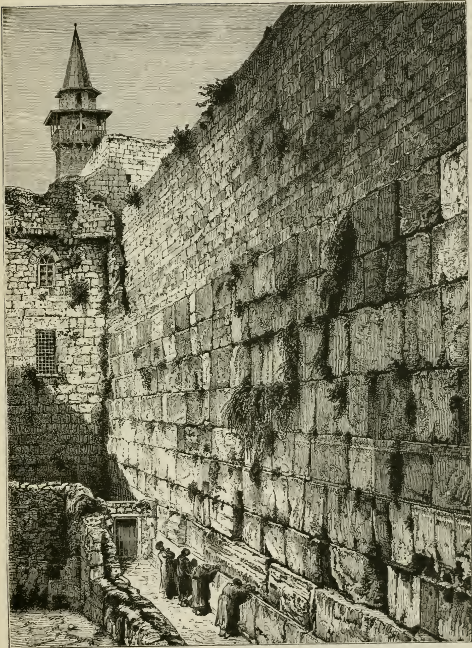
REMAINS OF THE TEMPLE WALL.—WAILING-PLACE OF THE JEWS.
